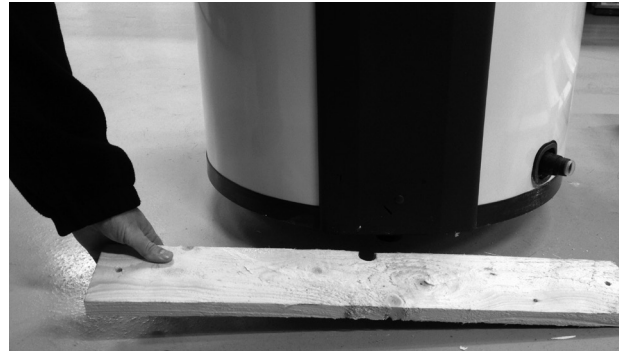
7. Removal of 1st piece of wood (can be released if product is tilted to one side).
