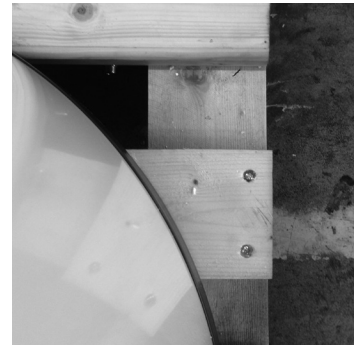
1. Screws to be removed (torx).
